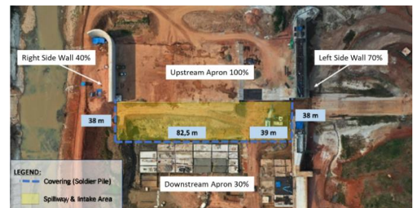
Figure 3 Actual condition of Margatiga Dam Project
