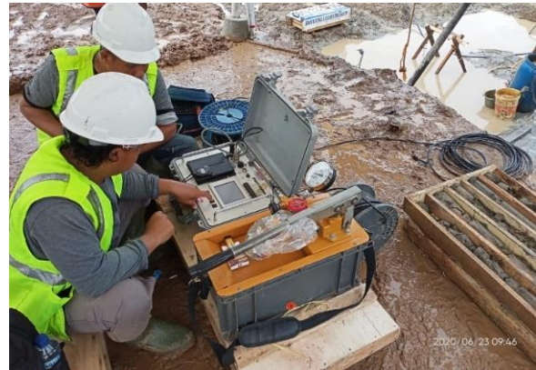
Figure 10 Pressure Meter Test in the spillway area of Margatiga Dam Project
