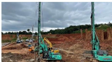
Figure 18 Documentation of boring activity at Margatiga Dam Project
