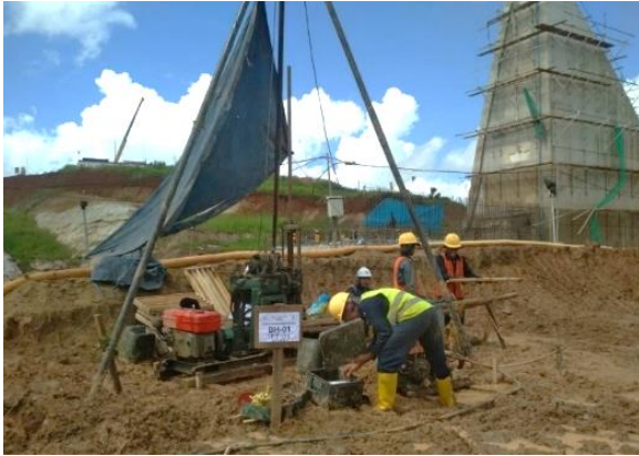
Figure 8 Standard Penetration Test in the intake area of Margatiga Dam Project
