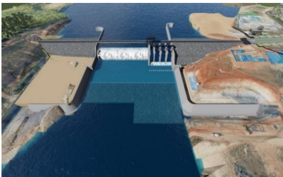
Figure 2 BIM 3D Model of Margatiga Dam Project
