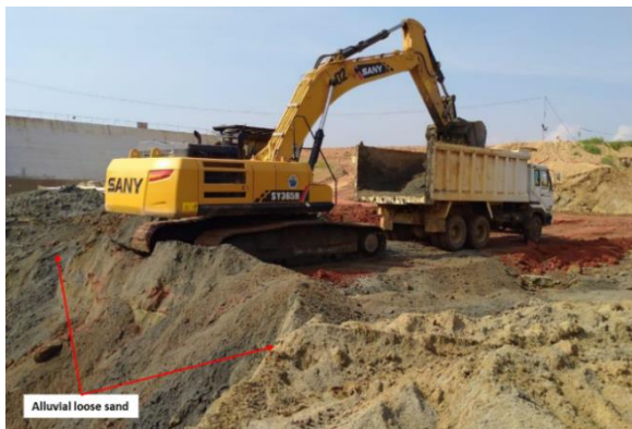
Figure 6 The condition of spillway area that dominantly consist of alluvial sand
