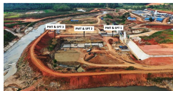
Figure 7 PMT & SPT location (view from downstream)
