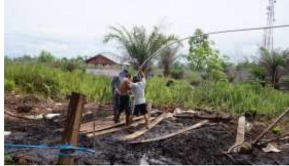
**Gambar 27** Pemasangan settlement plate Model fisik tipe C
