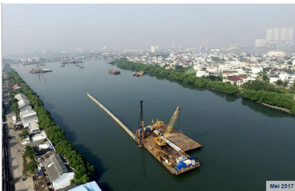
Figure 6 Dike construction area and their process in Muara Baru
